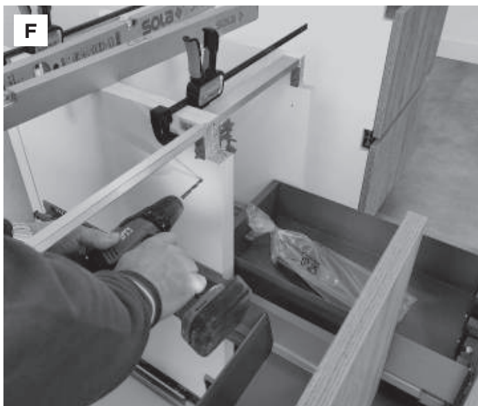
To unite Armony base units, pre-drill the panels. Use a drill with 5.5mm bit to complete the holes (F) (G).
