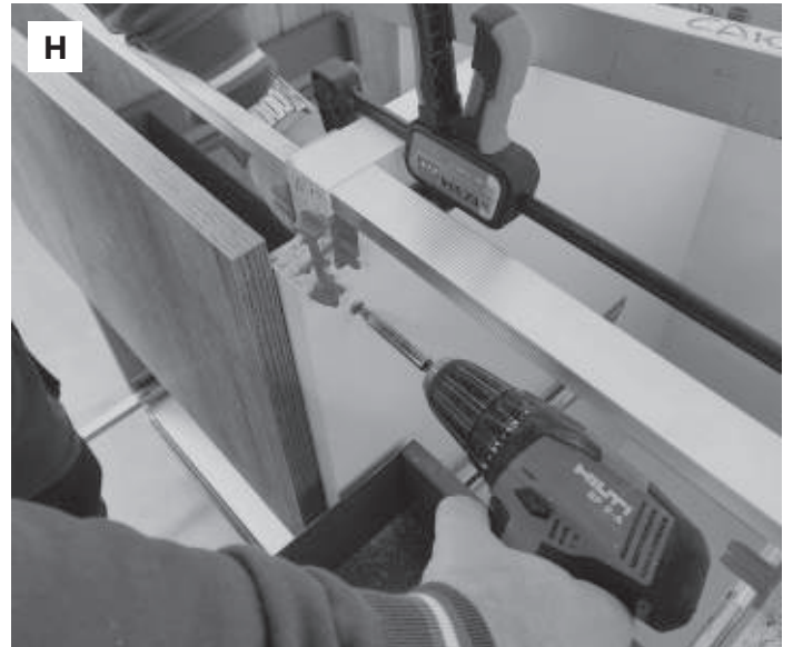
Using a mechanical screwdriver, lock the opposite side (H). Repeat for all drill holes: two for base units, two for wall units and three for tall units.
