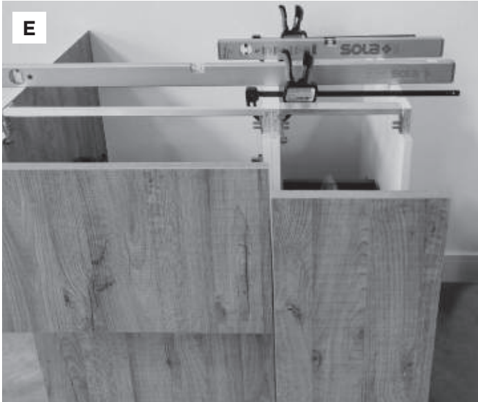
Join the bases with a clamp and check with a spirit level.
